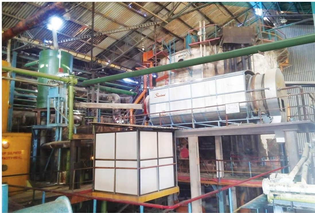
Figure no. 2: - Installation of Rotary Screen for hot juice screening
